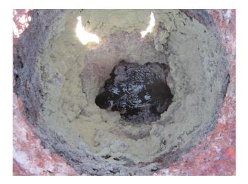
Severe H2S gas deterioration after multiple rounds of failed spray-on products
